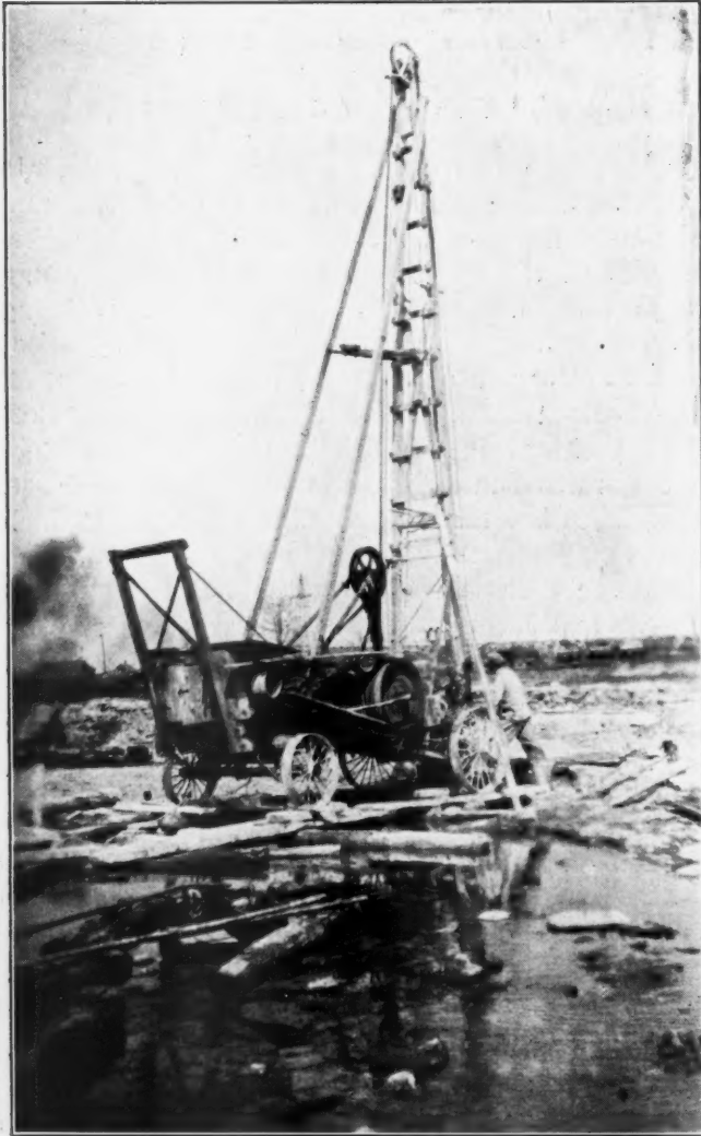
Close-up View of the Well Drill
